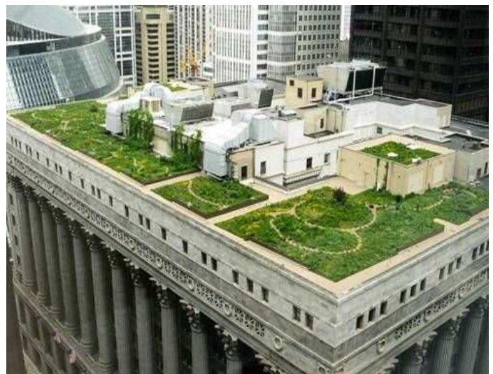
In 2001, a 20,300 square-foot green roof was installed atop Chicago's City Hall as part of Mayor Daley's Urban Heat Island Initiative. When compared to an adjacent normal roof, City Hall's green roof was nearly 100 degrees lower, and contributed to $5,000 in annual energy cost reduction, in addition to improving air quality and reducing stormwater runoff.
