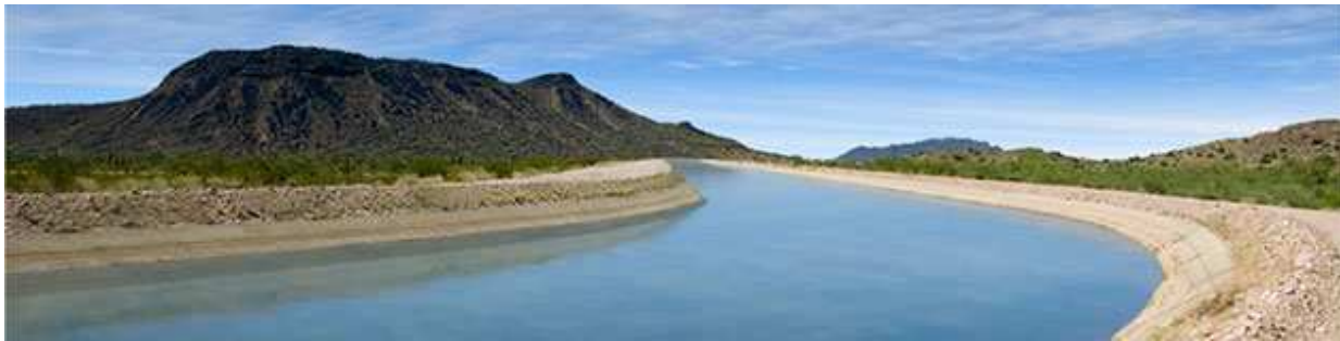
The Central Arizona Project is a 336-mile long system of aqueducts, tunnels, and pumping plants. Image credit: Central Arizona Project
