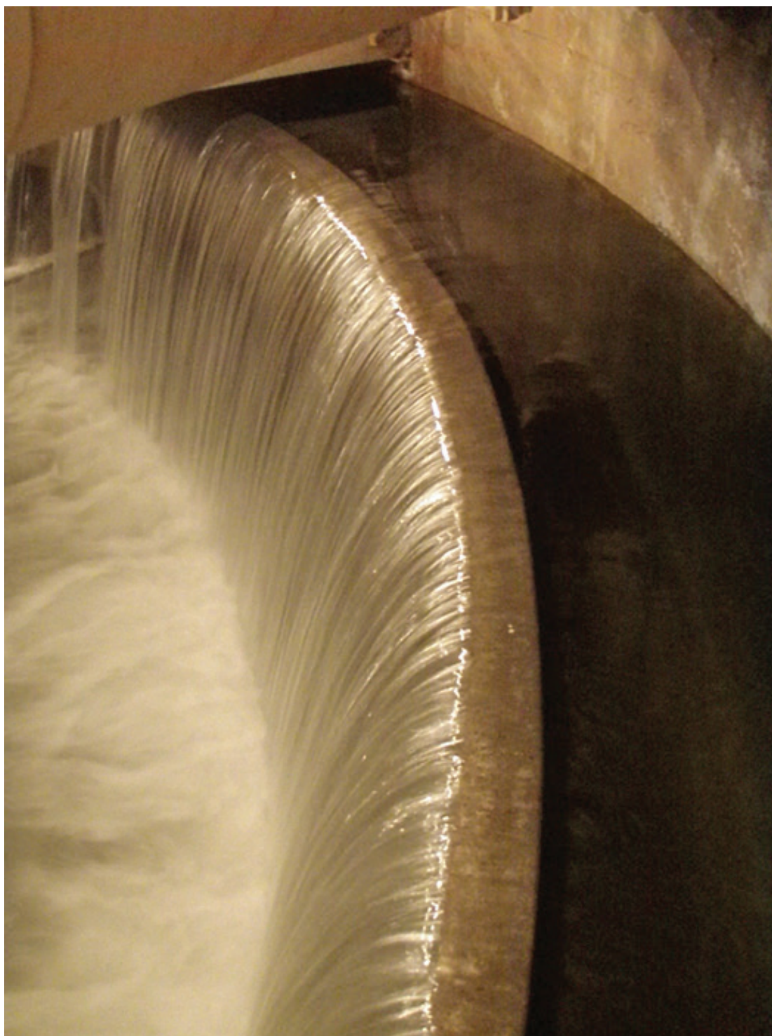
Figure 1. Salt water flowing over a weir and into a pump station.
