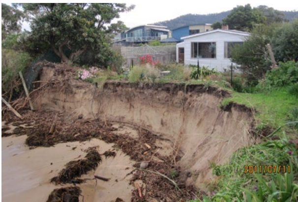
© Image Courtesy of CCC Figure 7: Dune erosion in July 2011 at Lauderdale, Tasmania
