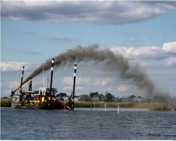
Figure 6. Spraying of dredge spoil to raise elevation of marsh. (Credit: U.S. Army Corps of Engineers)
