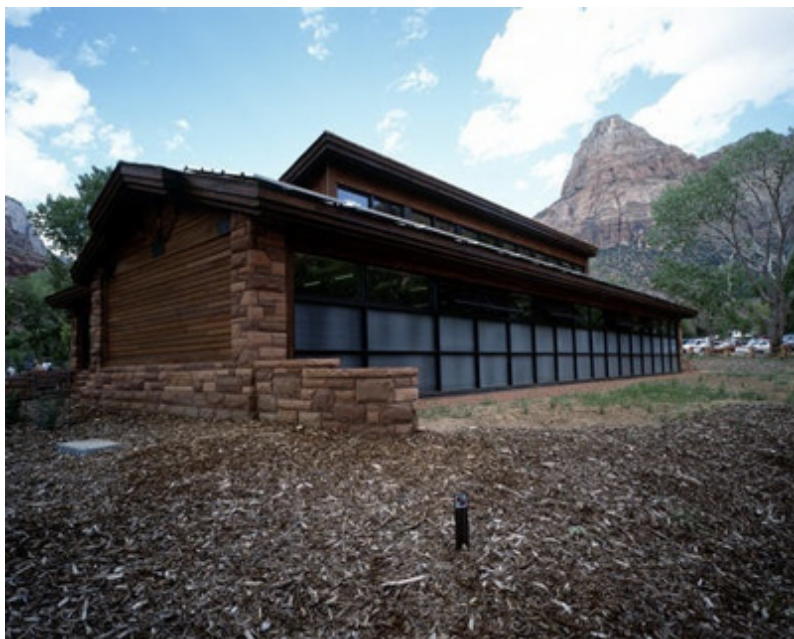
Zion's Visitor Center showing Trombe wall and clerestory windows.
