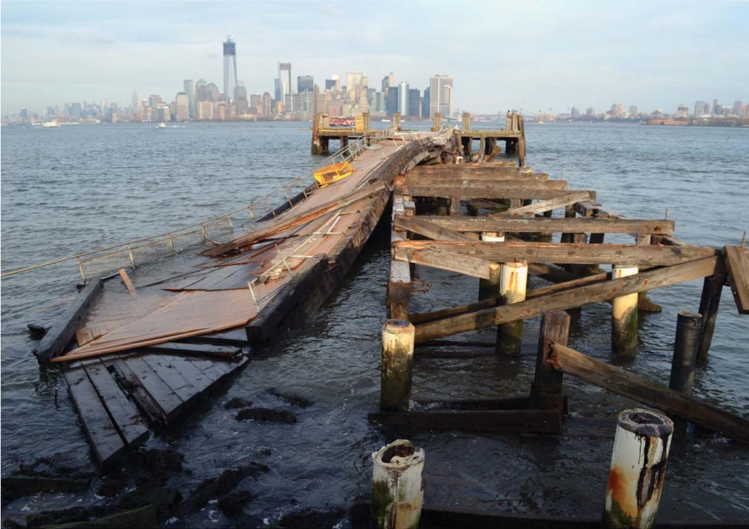
**Figure 2.** Damaged by Hurricane Sandy in November 2012, this dock at Liberty Island in New York Harbor is a stark reminder of the combined effects of sea-level rise and storm surge. As sea levels increase, severity of potential storm surge also increases. Storm surge is often overlooked by managers planning for the impacts of sea-level rise.
