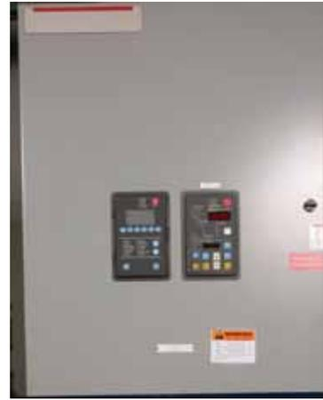
Upgraded Multi-Function Relay, Metering, and Controls
