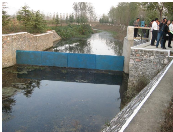
Figure 3: Water harvesting using flip gates, canals, and on-field storage (World Bank, 2011).
