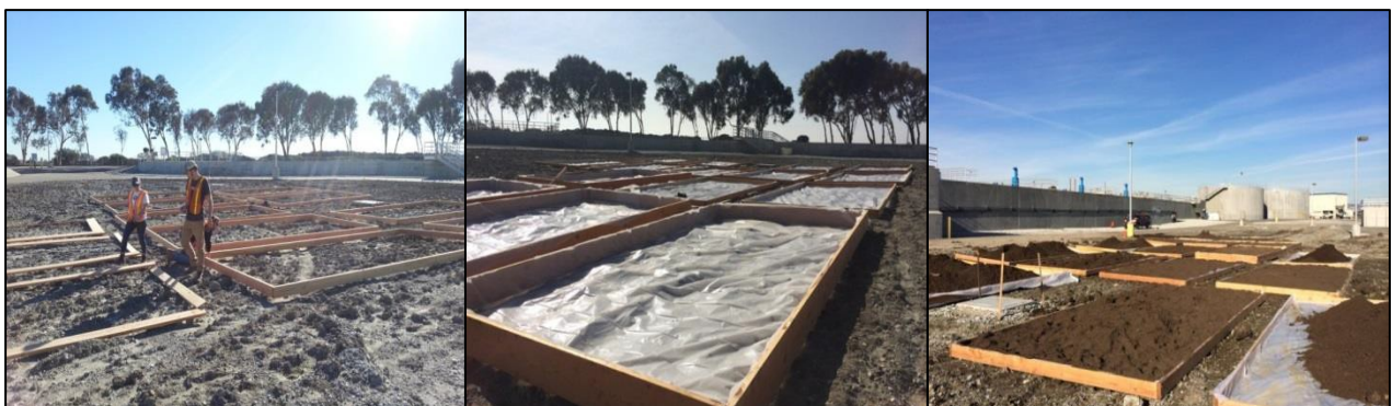
Figure 4. Raised bed construction at the Oro Loma Wastewater Treatment Site.
