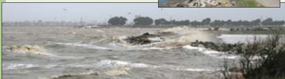
2005 storm overtops Hayward Shoreline levees. Inset: Same levee after storm. Lower photo: Mark Taylor
