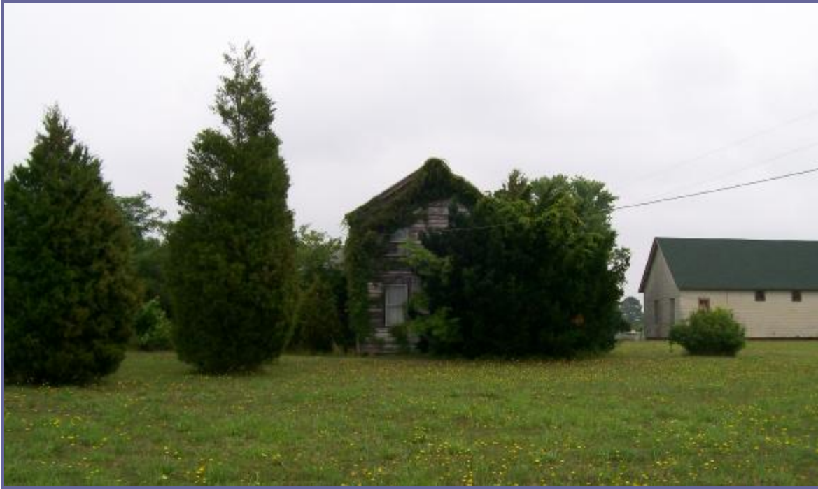
Abandoned property on Elliott Island Road.
