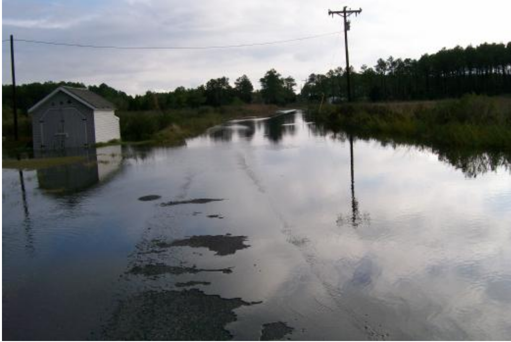
Aisquith Island Road during a spring high tide and strong south winds. The tide of Charles Creek was one foot above mean high water elevation. Crapo, Maryland October 27, 2007
