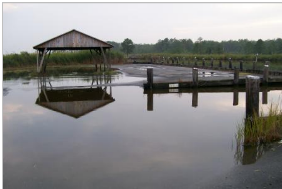
Boat ramp, pavilion, and parking lot inundated by spring high tide. Transquaking River at Bestpitch Ferry Road. October 27, 2007
